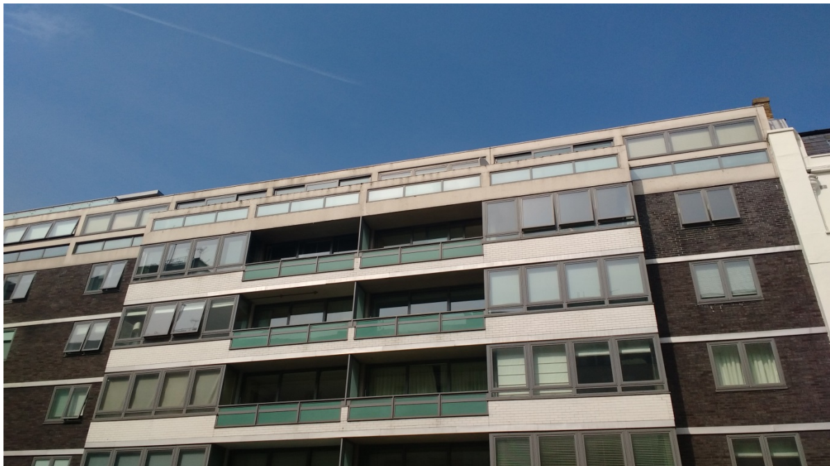
View of Flat 25 from Lowndes Street
